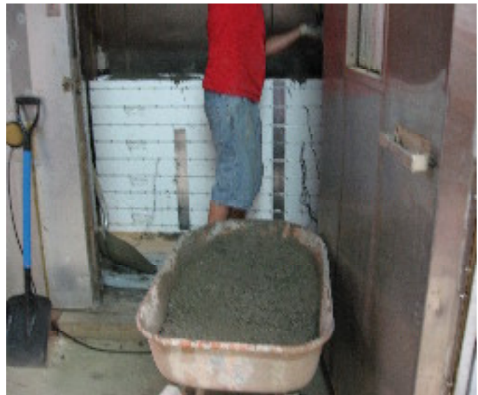
The construction of the concrete wall with the Permaform
