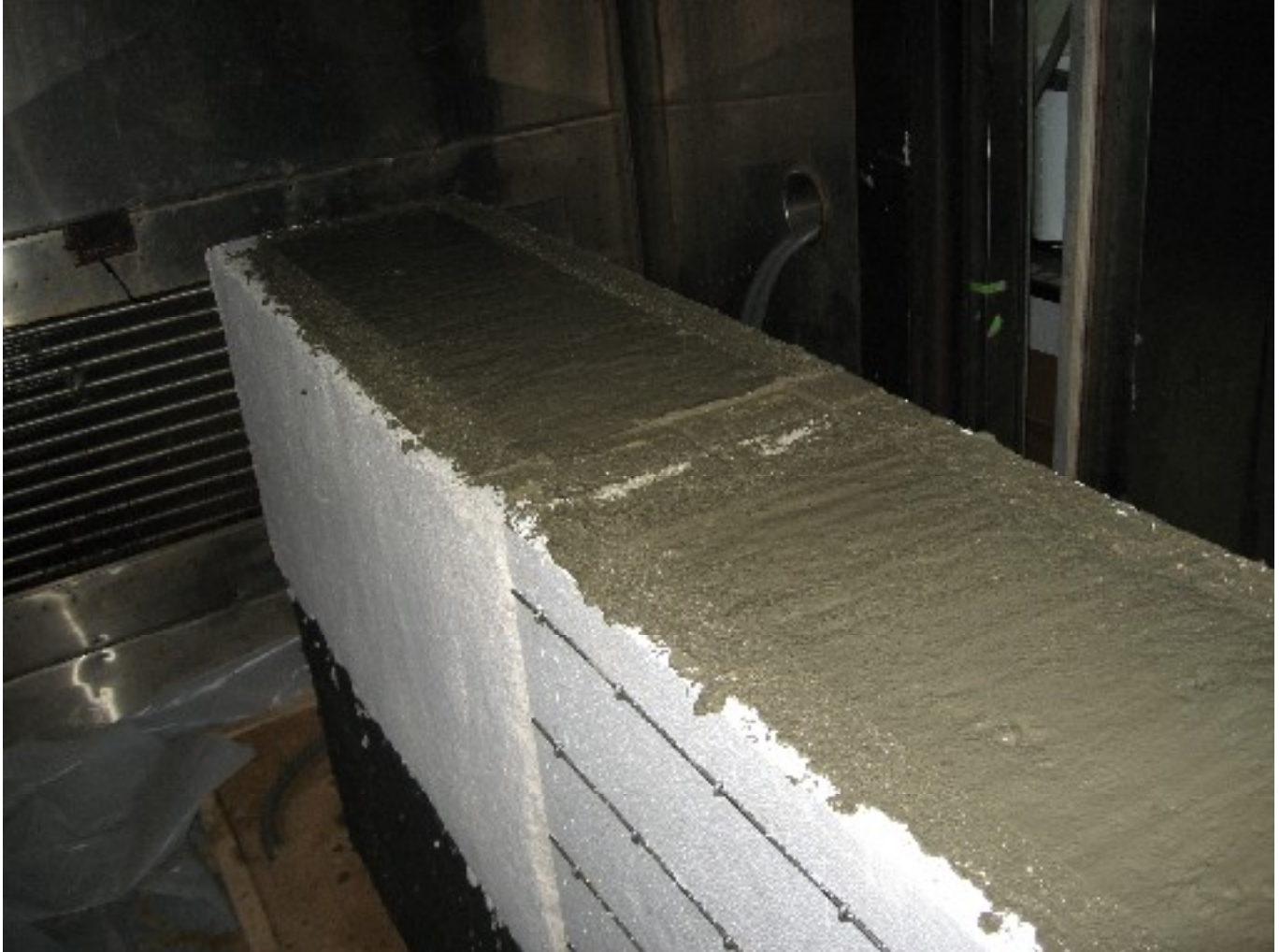
View from inside of the chamber, bare Permaform wall on the right, Stucco coating on top left, and rubber coating on the bottom left
