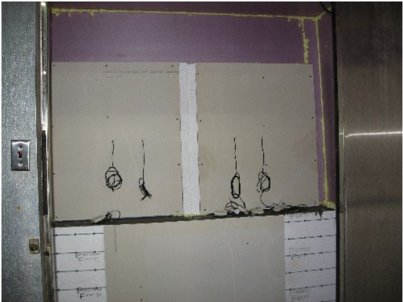
The upper portion of the wall in this picture contains the fiberglass insulations
